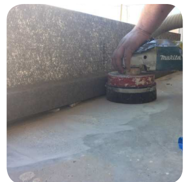
Protect edges from damage
